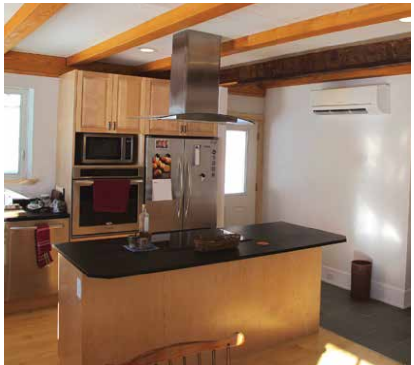
Left: The author has a woodstove for backup heat. Right: The indoor unit of his home's air-source heat pump hangs on the far kitchen wall.
