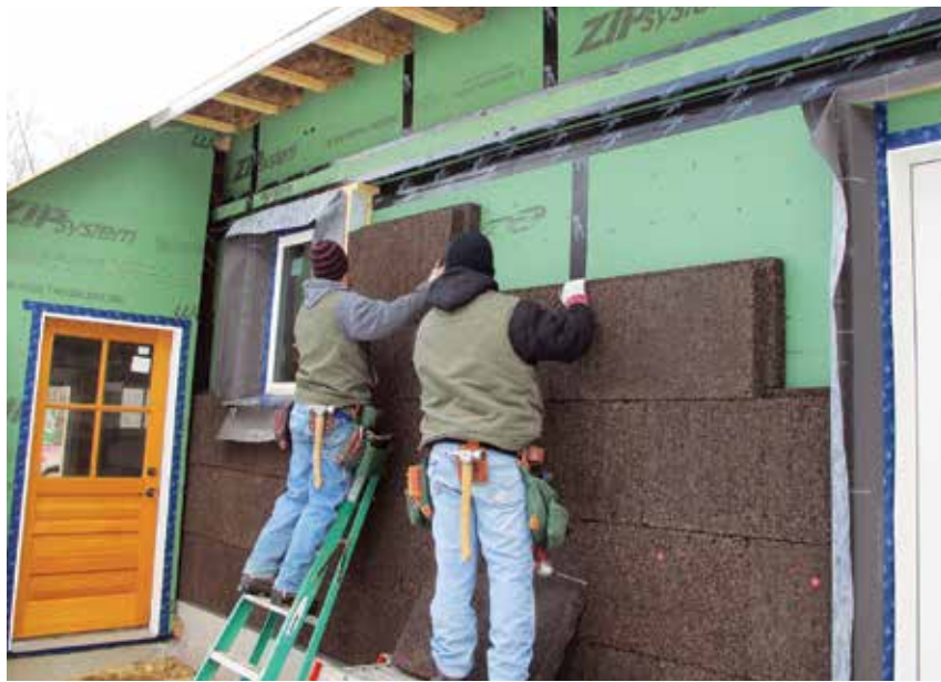
Cork insulation is part of the super-insulation strategy that allows the author's family to heat their home with an 18,000-Btu-per-hour air-source heat pump.
