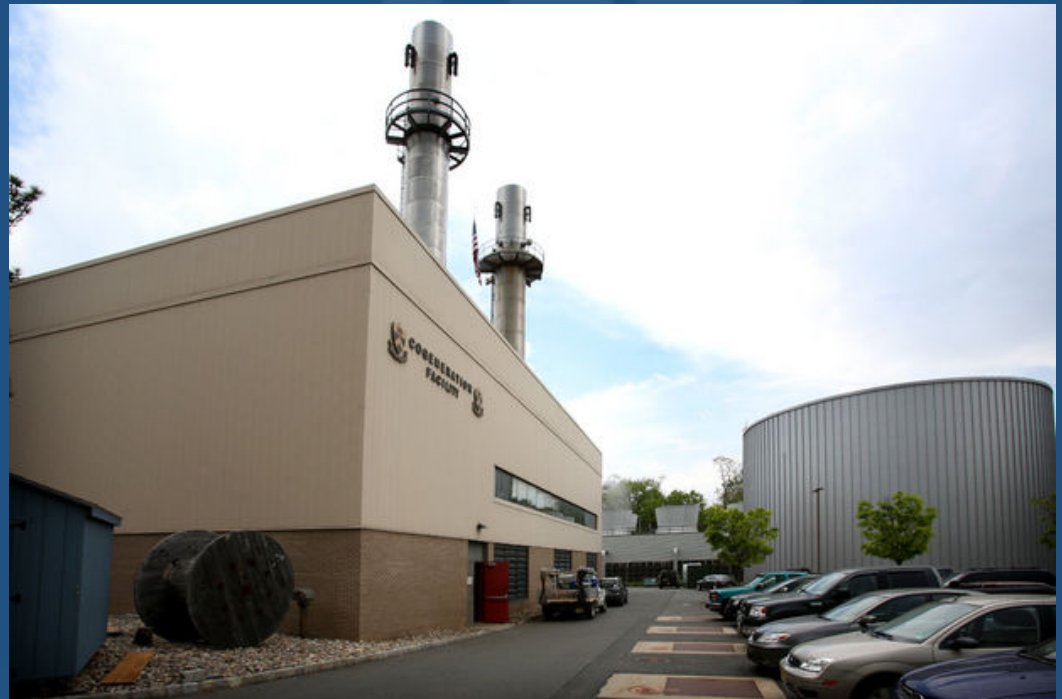
Princeton University CHP plant showing 2.6-gallon chilled water tank – photo: Martin Griff, The Times of Trenton
