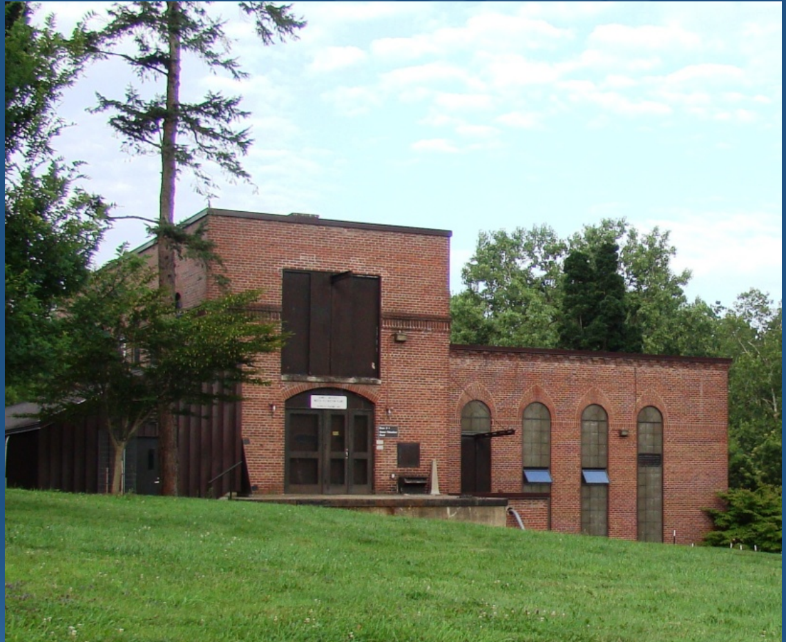
Cornell water filtration plant Photo: Cornell
