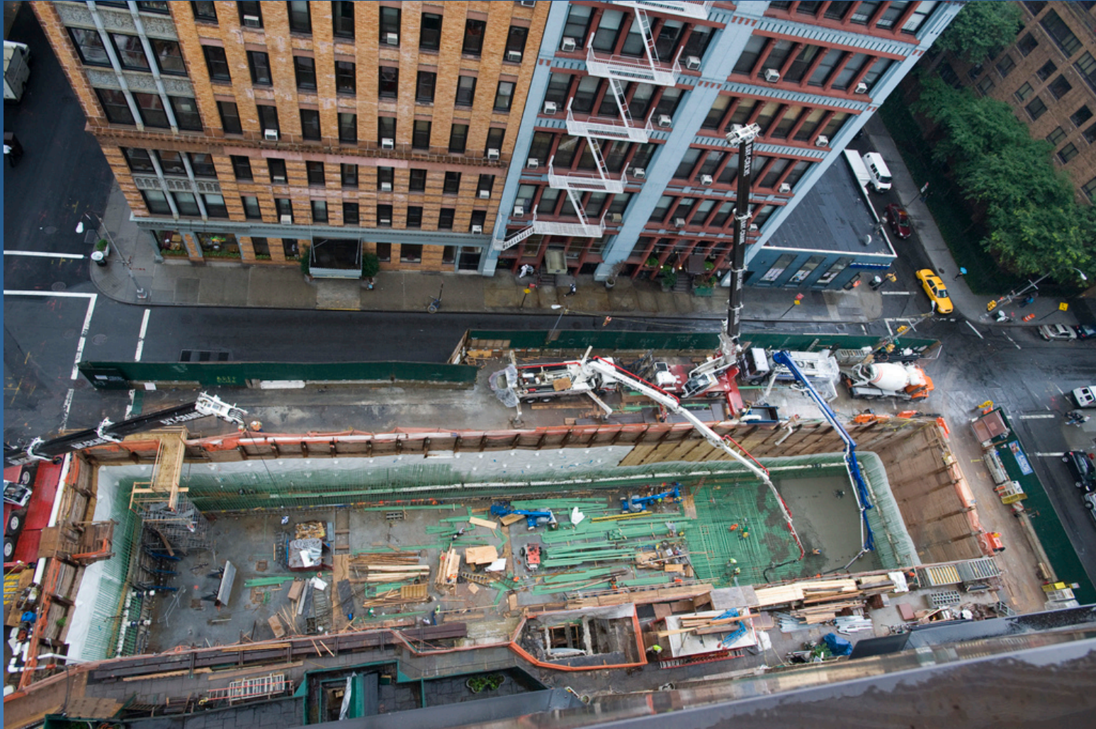
CHP plant being built under what will be Mercer Plaza – photo: New York University
