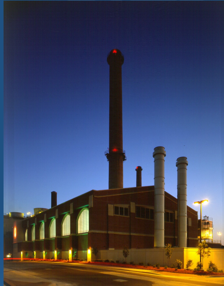
CHP plant serving the Univ. of Missouri, Columbia – photo: Assassi Productions
