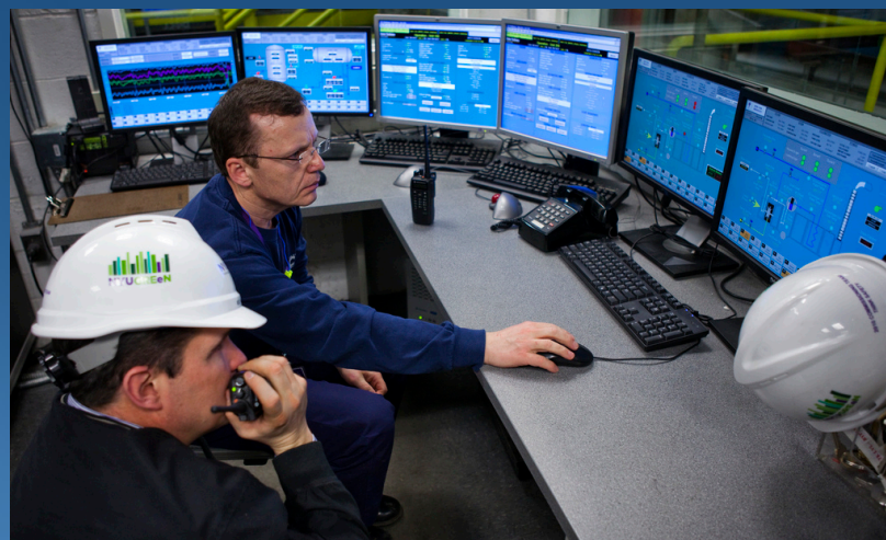
Control room Photo: NYU
