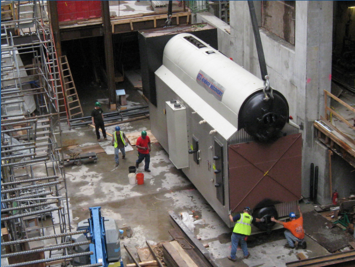
Energy recovery unit Photo: NYU
