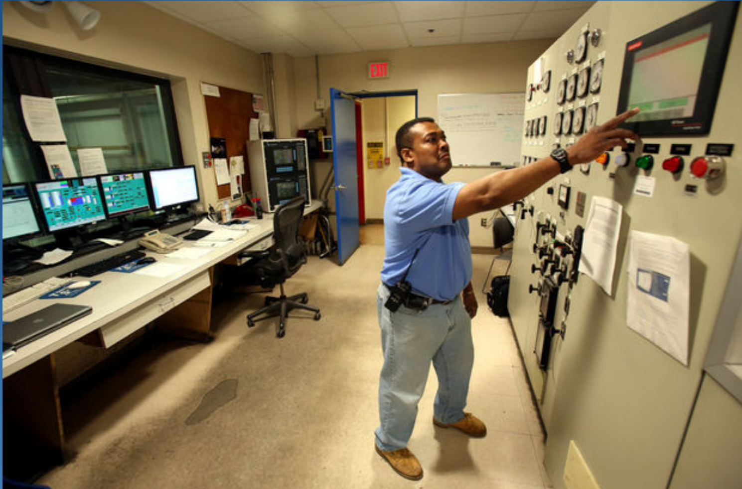
James Thompson of Princeton University Facilities synchronizing the power output from the CHP plant to the PSE&G utility grid – photo: Martin Griff, The Times of Trenton
