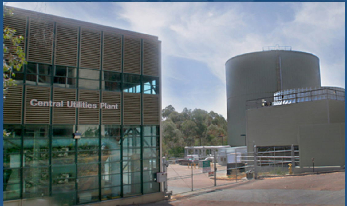
CHP plant serving the UC San Diego campus – photo: Rhett S. Miller, UC Regents
