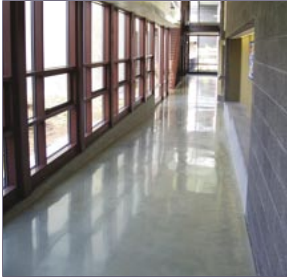
Polished, densified concrete, such as this installation at the Benjamin Franklin Elementary School in Kirkland, Washington, offers a highly durable, low-maintenance flooring option for schools.
