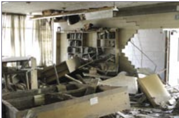
Damaged wall and furnishings in the library of the Alfred Lawless School, May 2006.
