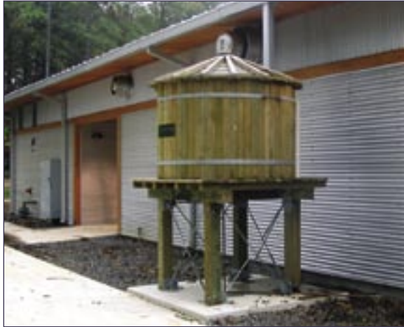
This 700-gallon cistern stores rainwater for the Camp Aldersgate Commons Building in Little Rock, Arkansas.
