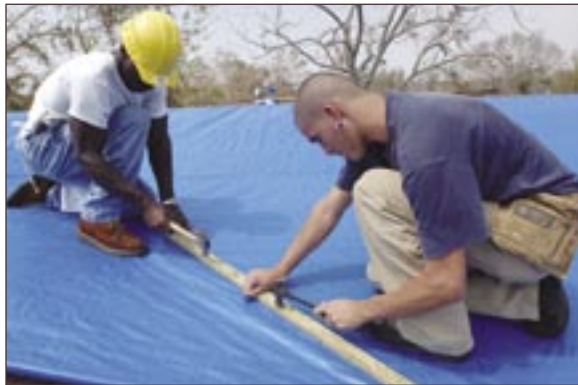
A construction crew from Mobile, Alabama, installs a tarp on a roof in Biloxi, Mississippi.
