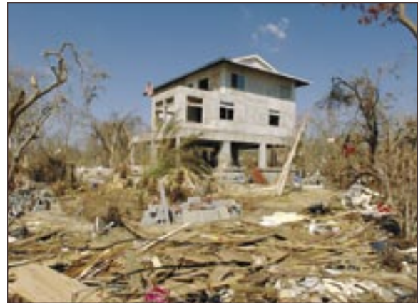
Mississippi resident Scott Sunberg in Pas Christian is building a steel reinforced concrete house to minimize damage from hurricanes. Still under construction, his was the only house left standing in the neighborhood after Hurricane Katrina.
